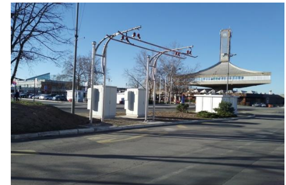
AC/DC Chargers on Terminal: Gale Muskatirovic, sport-center 2x400 kW
